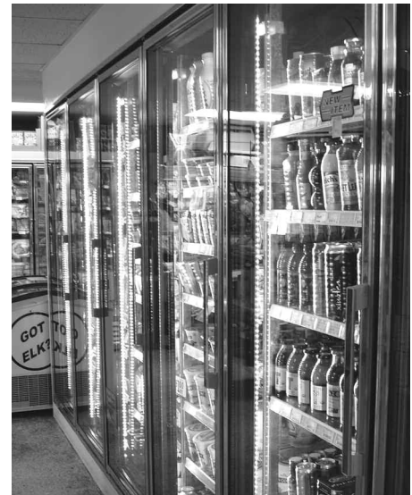
New LED lights
